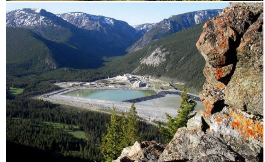
EAST BOULDER MINE (Sibanye-Stillwater)
